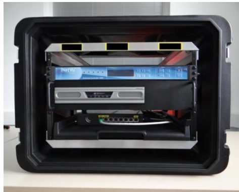
Fig.2. Devices: Mikrotik, iDirect X5 and Antenna Controller Unit.
