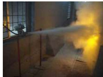
Fig. 20. fire suppression control valve with 80% opening.
