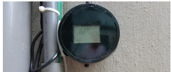
Fig.15. Deploying the Smart Water Meter in a Real Condition
